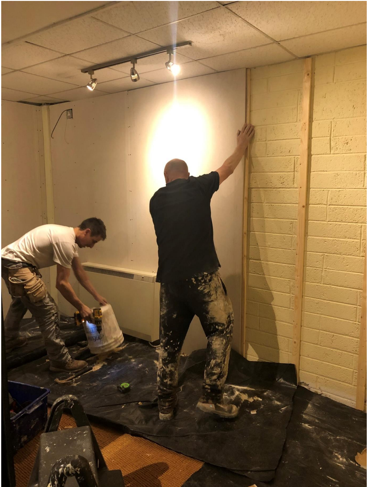
Figure 15 Plastering the upstairs room
